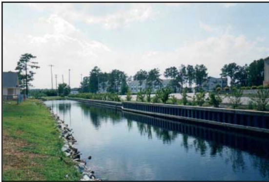
Trinity Presbyterian Church Installation - Surfside Beach, South Carolina
