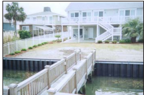
Residential Completed Installation - Wrightsville Beach, North Carolina
